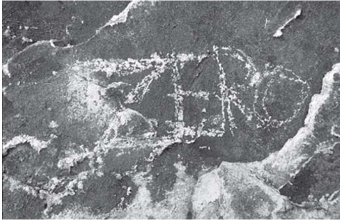
Figure 3. This is an unusual combination of natural and man-made deterioration. Here, the scratched graffito "ZERO" has been highlighted by preferential efflorescence of natural soluble salts in the scratches. Pictograph Cave State Historic Park, Montana.
